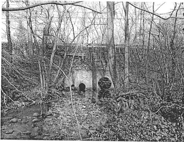
Storm Pipes Discharging from Under White Horse Pike
